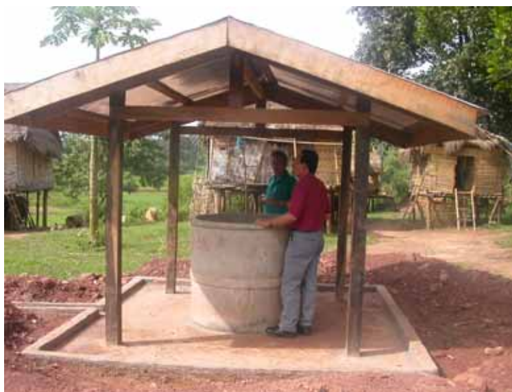
Dug well near completion
