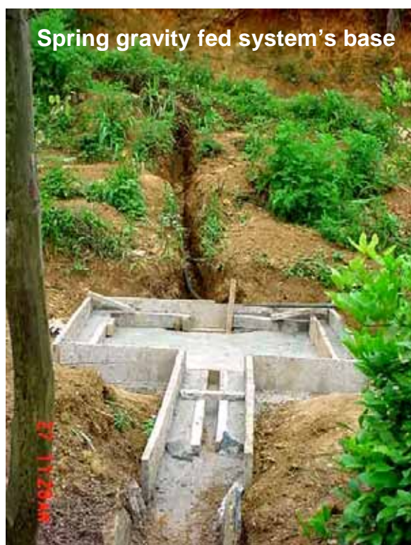
Construction of Spring gravity fed system in Huaphanh Province
