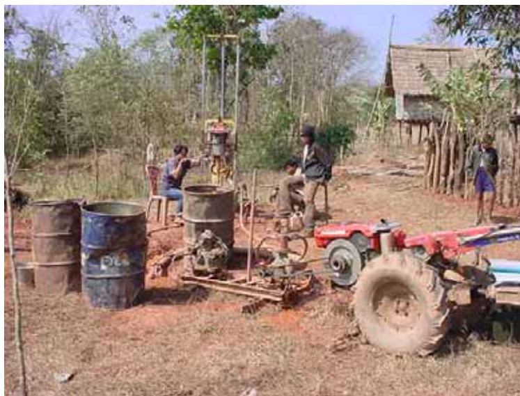
Drilled well and local contractor
