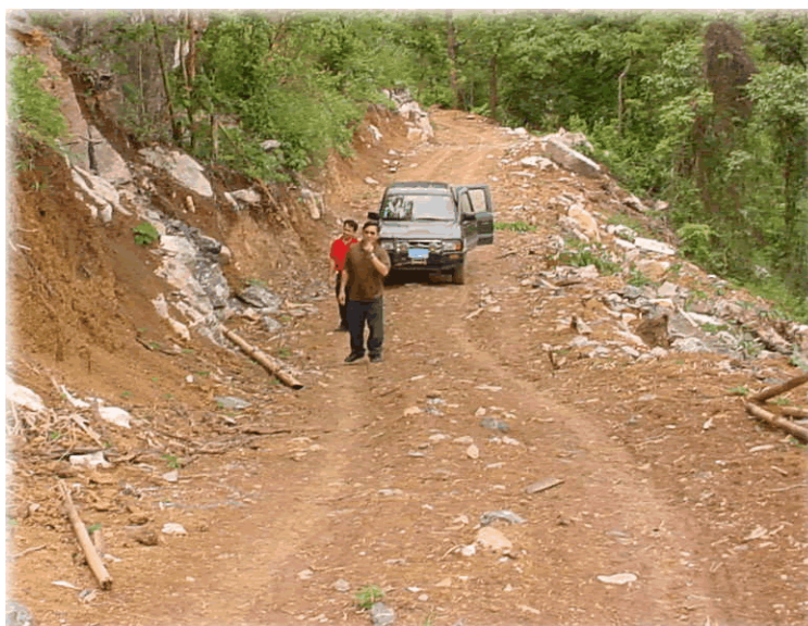
PRF staff checking the quality of road construction in Xamtay District
