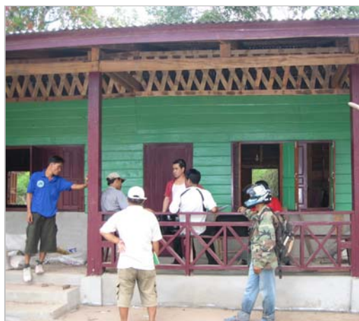
Dispensary Construction Toumlan district, Saravanh Province
