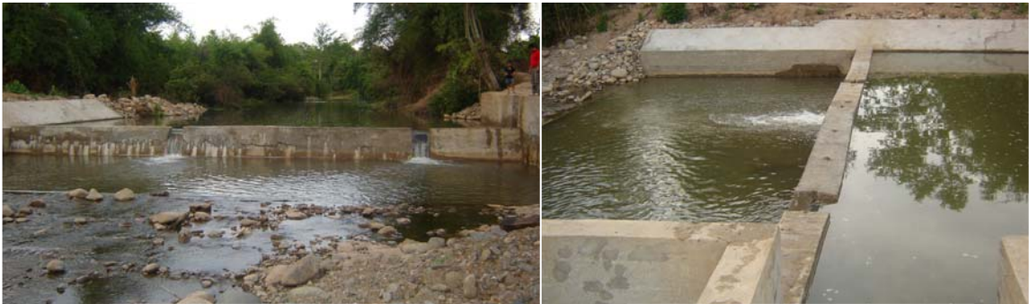
Irrigation Dam, Kham district Xiengkhouang province
